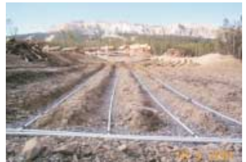
Pressure-dosed drainfield laterals in trenches ready for burying
